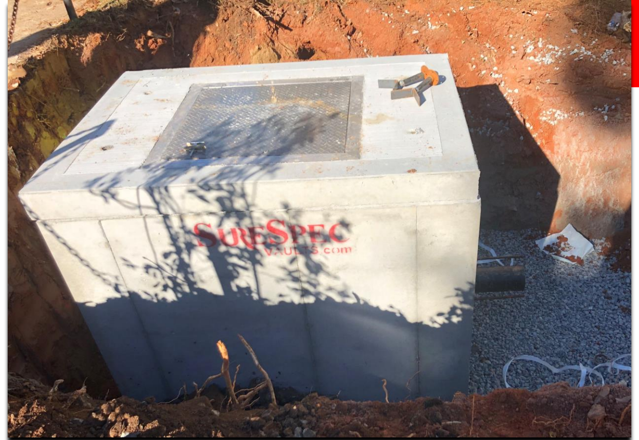
Water Meter and Vault Installed
