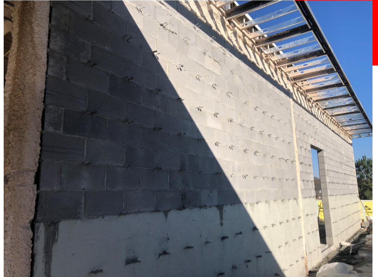
4 th Floor Exterior CMU walls Complete
