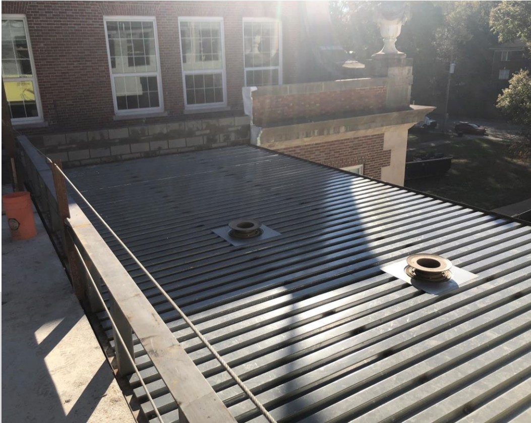
Decking and Roof Drains Installed at Bridge, Ready for TPO Roof
