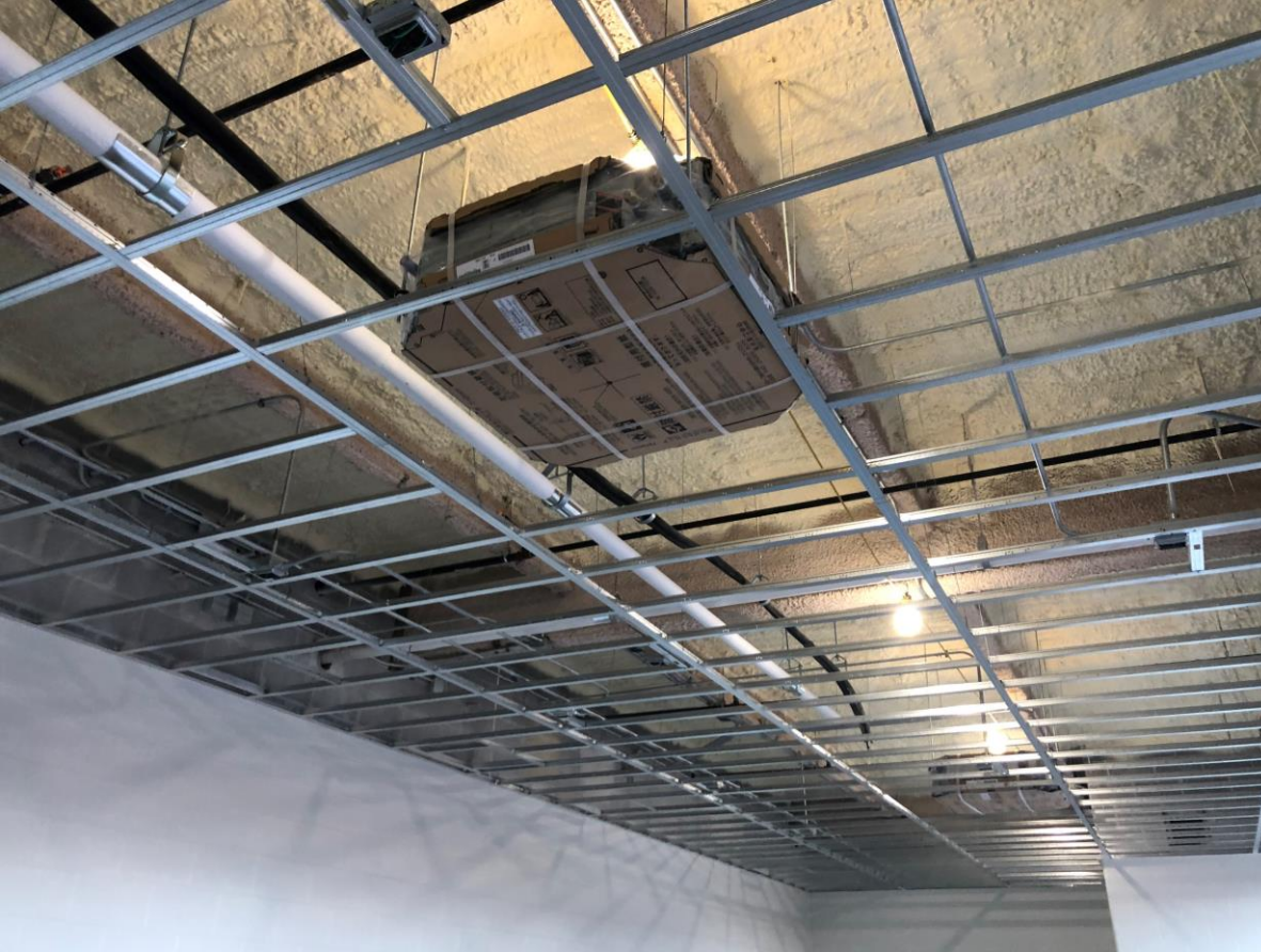
VRF Cassette Units Installed 1 st and 2 nd Floor of New Addition
