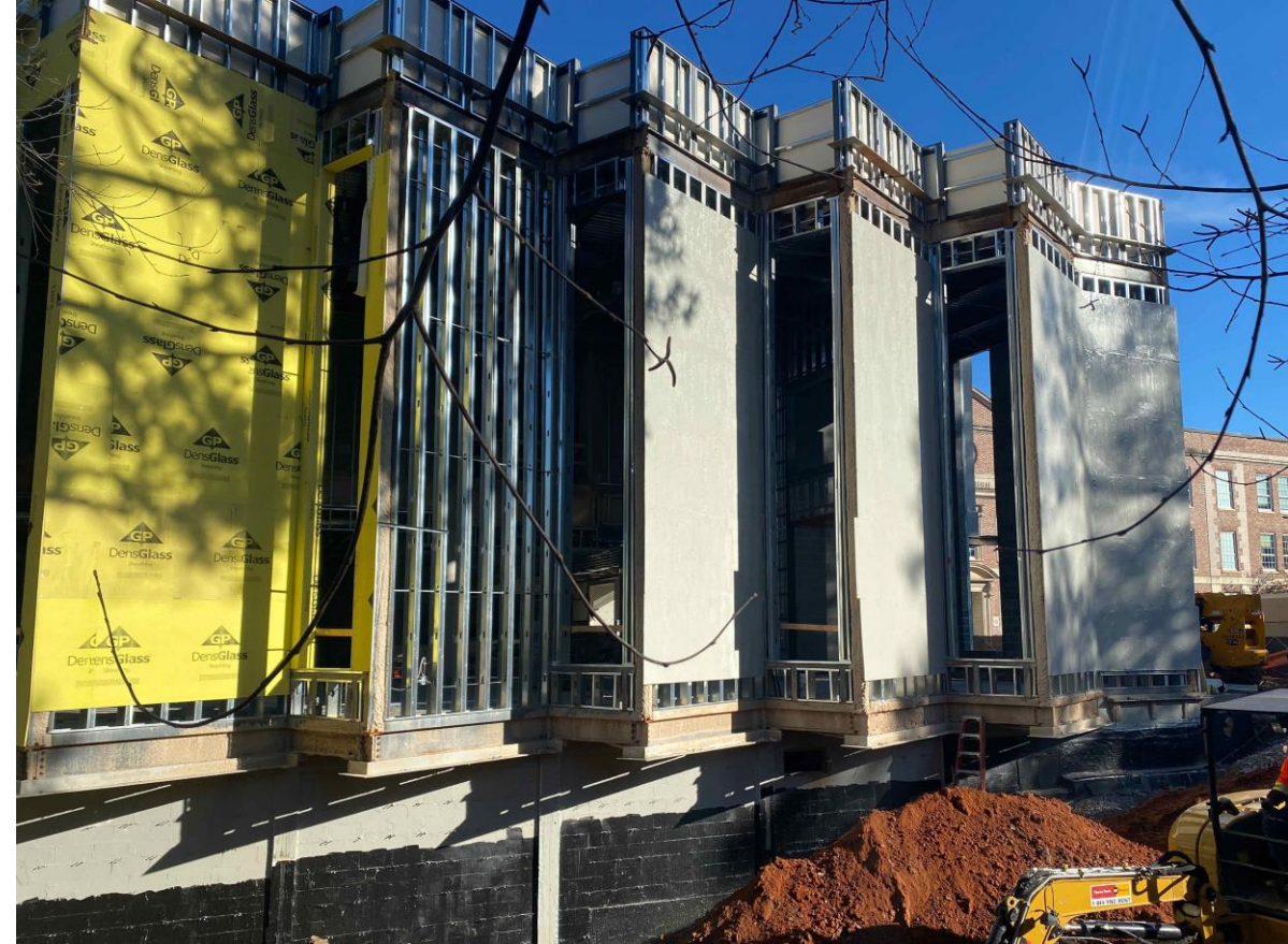
Exterior Sheathing and Waterproofing Progress West Wall of New Addition
