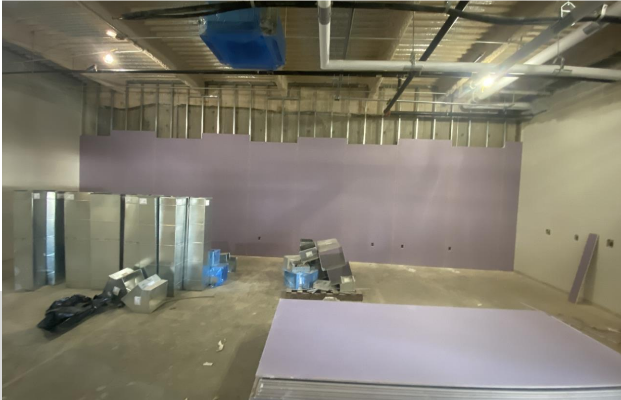
Gypsum Board Installed
